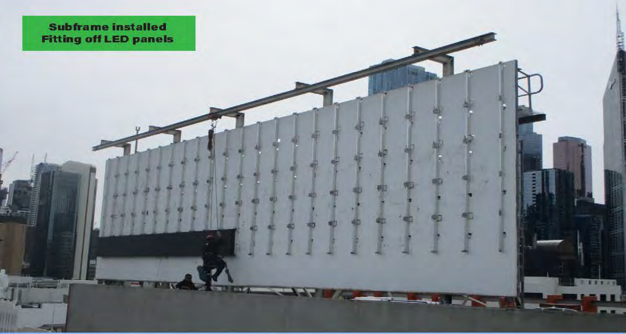
Install final LCD Panel
